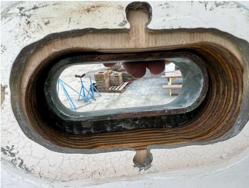
Dry fit and then epoxied into place
